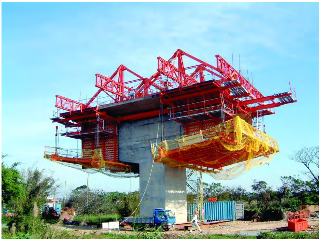
Figure 2.10: Travelling Formwork
